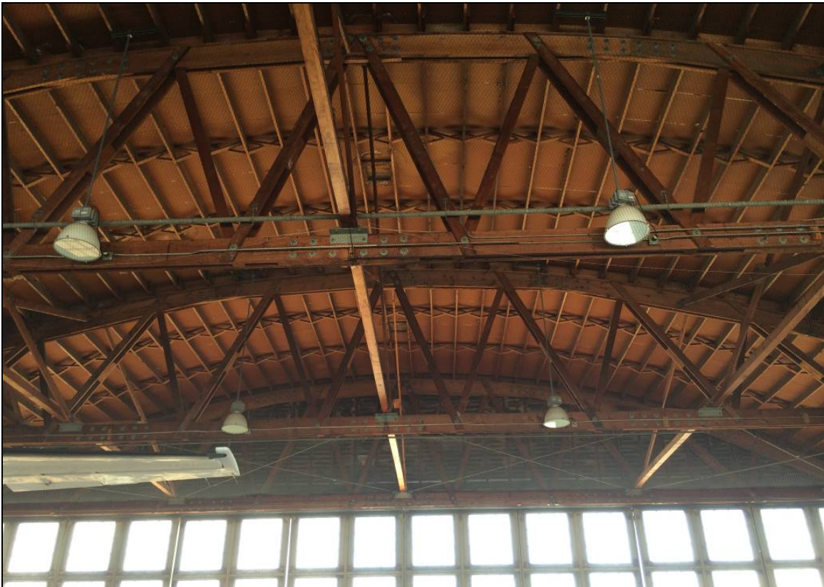
Figure 4-13 Interior view of the closed-arch trusses in Hangar No. 1.
