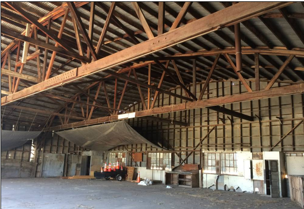
Figure 4-3 Interior view of two closed-arch trusses and the north (rear) façade of Building 248.
