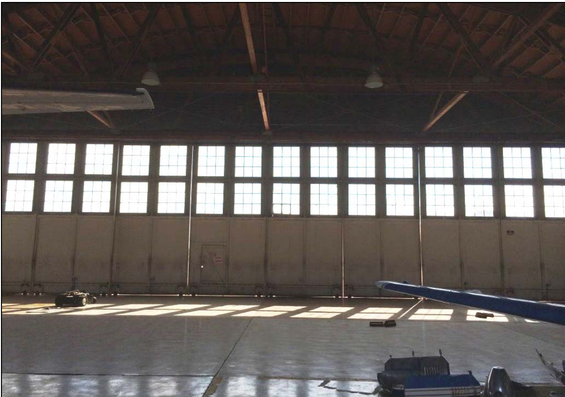
Figure 4-15 Interior view of the sliding hangar doors in Hangar No. 1.
