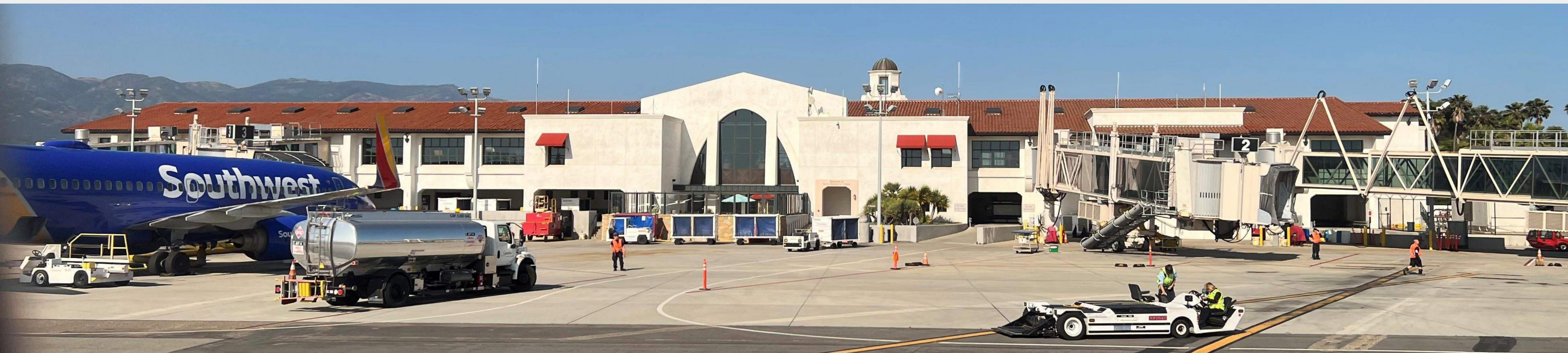
Air Side West Elevation
