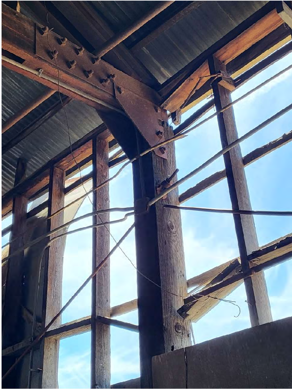
BUILDING 248 – BOWSTRING TRUSS WESTERLY CONNECTION 1
