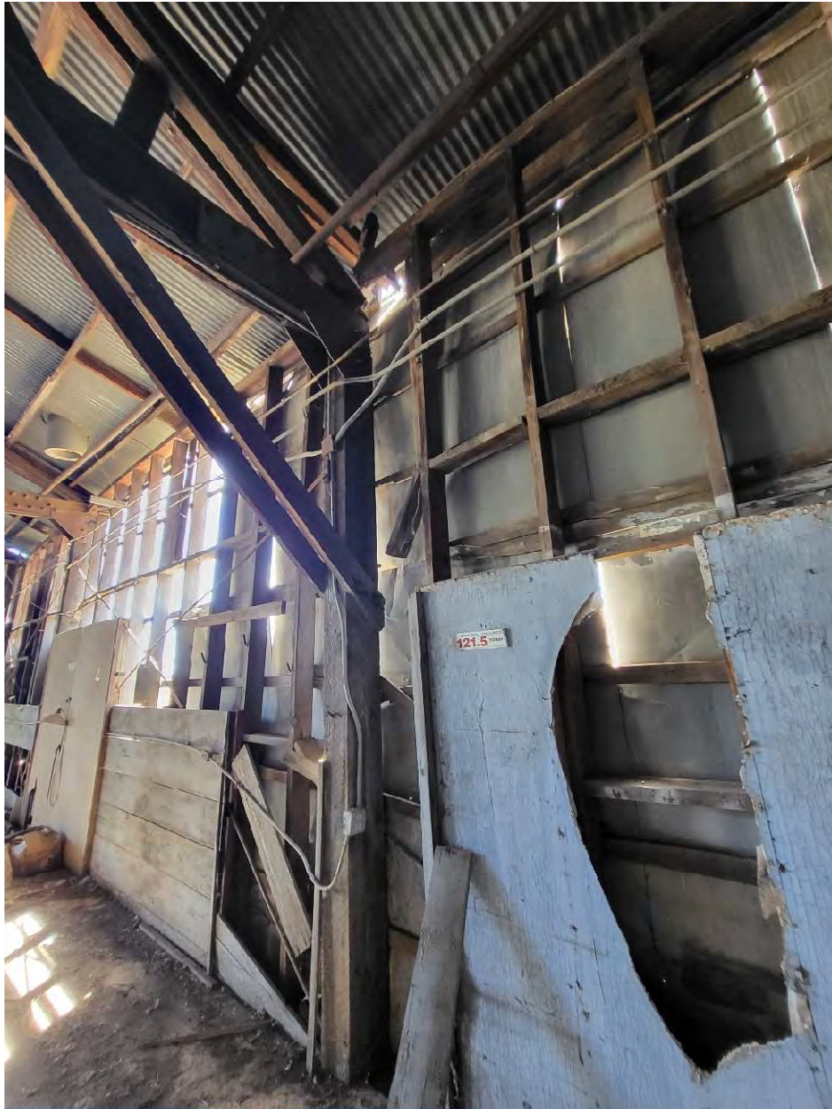
BUILDING 248 – BOWSTRING TRUSS WESTERLY CONNECTION 2
