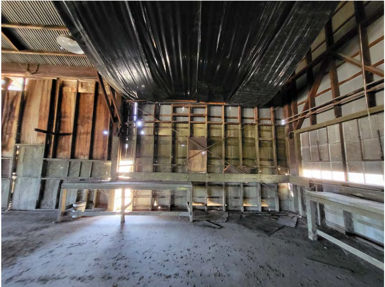
BUILDING 249 – ROD DIAGONAL BRACES
