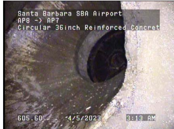
605.60ft Manhole / AP7
