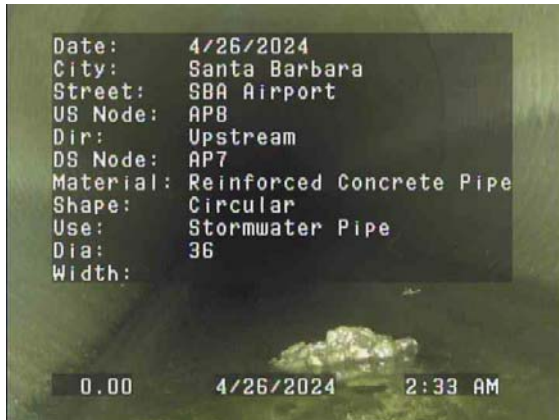
0.00ft Manhole / AP7
