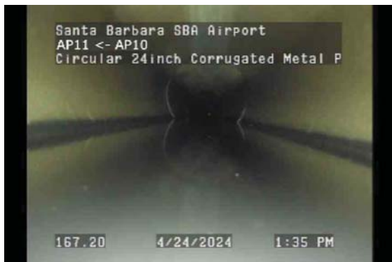
167.20ft Miscellaneous Material Change, Reinforced concrete pipe / RCP
