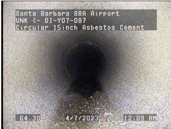
64.30ft Deposits Settled Other, 5% of cross sectional area from 5 o'clock to 7 o'clock / Debris
