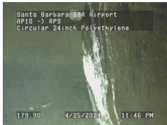
179.90ft Miscellaneous General Photograph from 7 o'clock to 11 o'clock
