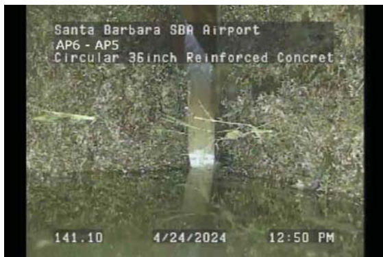
141.10ft Discharge Point / AP5
