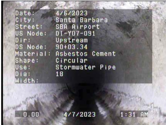
0.00ft Catch Basin / 90+03.34
