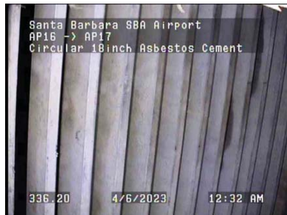
336.20ft Catch Basin / AP17
