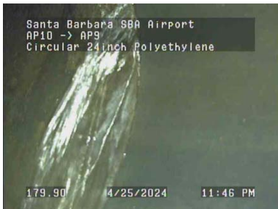
179.90ft Miscellaneous General Photograph from 1 o'clock to 5 o'clock
