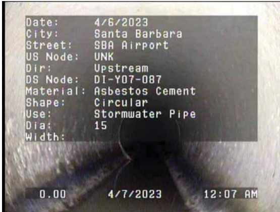
0.00ft Catch Basin / DI-Y07-087
