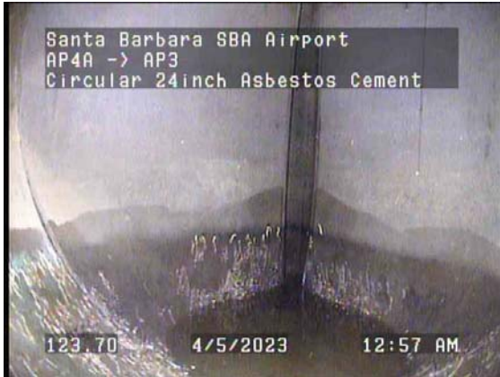
123.70ft Discharge Point / AP3
