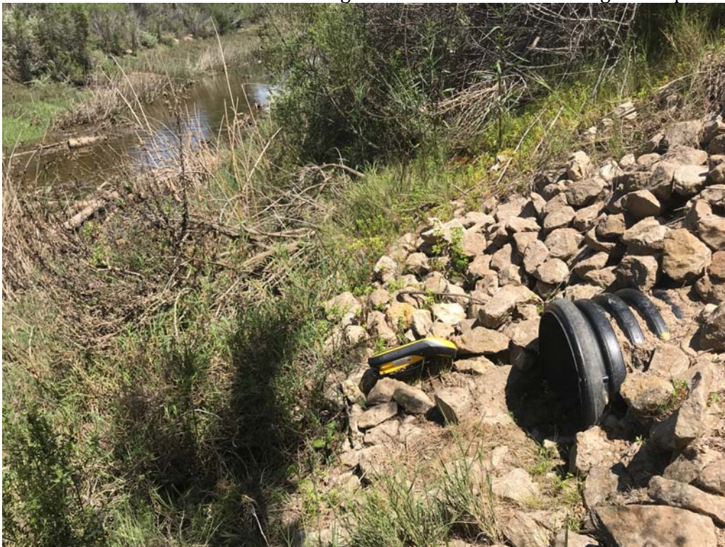
Photo 18. One of the drain outfall structures along Carneros Creek.
