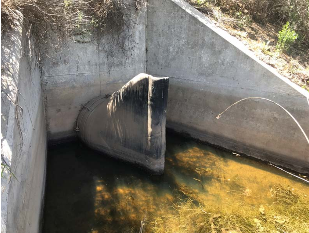
Photo 19. Larger drain outfall structure with one way flow control to prevent water from backing up into the site during high flow and rain events. Note pipe is partially submerged in April 2018.
