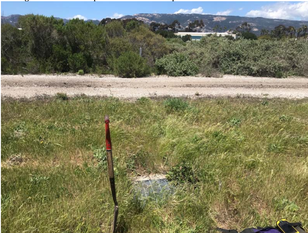
Photo 16. One of the drain inlets present in the study area that direct surface runoff to Carneros Creek, which is present just on the other side of the unpaved perimeter road.
