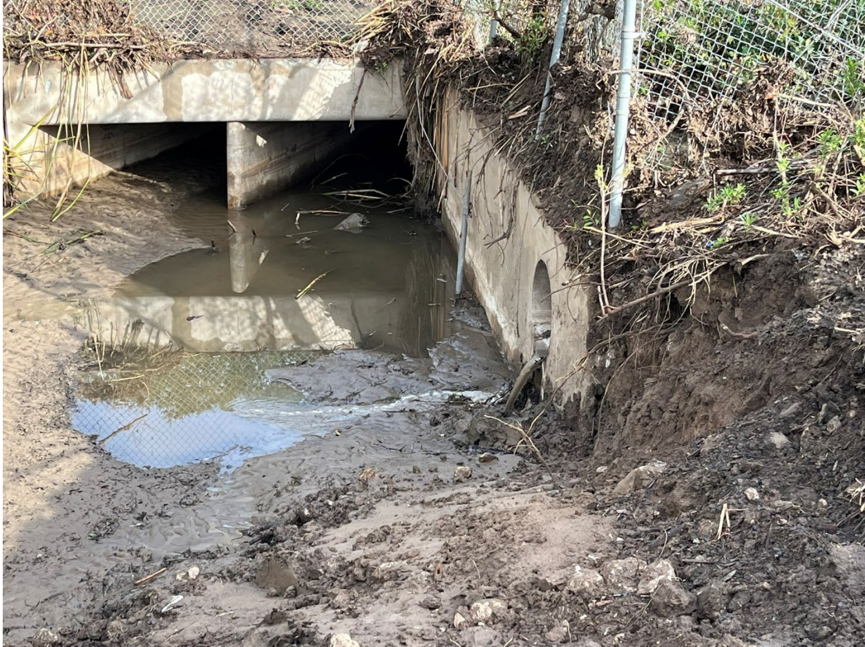
Figure 23. Firestone Road Drainage Channel Box Culverts under Firestone Road at Outlet to Carneros Creek
