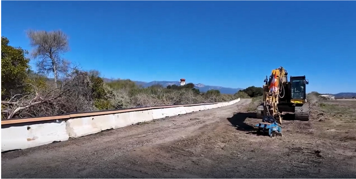
Figure 10. K-Rail Deployed Along the Service Road South of Carneros Creek in 2025
