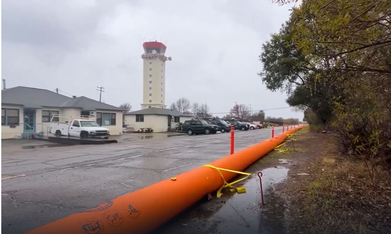
Figure 8. Inflatable Tiger Berm Deployed Along Firestone Road in 2025
